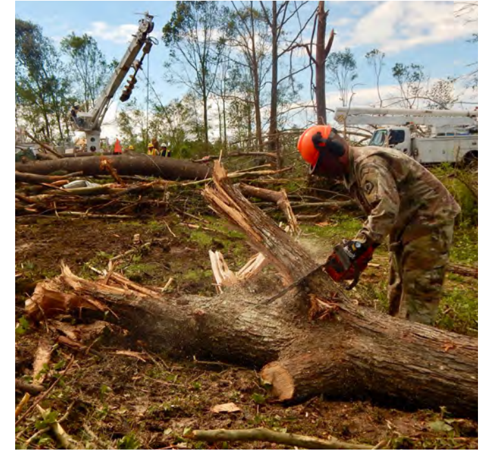
Sgt. William Grayson, a mechanic with Field Maintenance Shop 9 in Florence, works with emergency responders to remove uprooted trees on Sgt. 1st Class John Paul “JP” Wallace’s property in Morton, April 19. Grayson, along with fellow Mississippi Army National Guard maintainers were present to help Wallace recover from an EF-2 tornado that damaged his home the day before.
